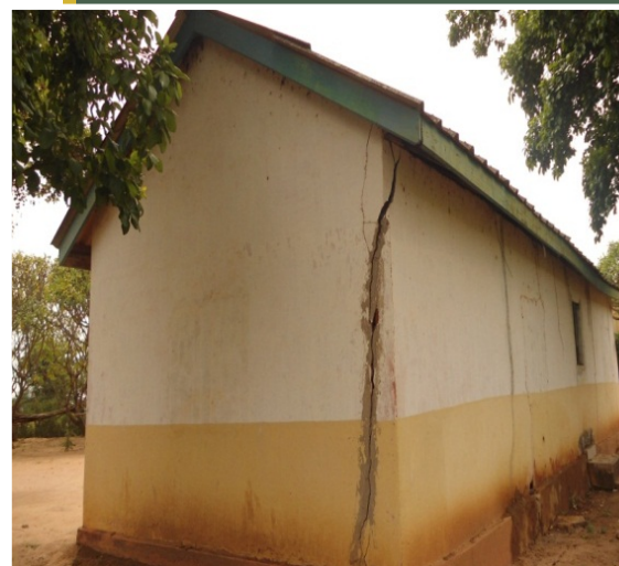
The dangerously cracked walls of Makueni Law Courts.
